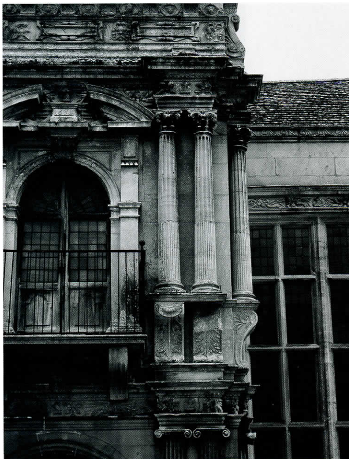
19. Upper level of the hall porch, Kirby Hall.
