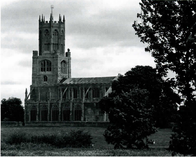
1. Fotheringhay church (Northamptonshire) from the south-east.
