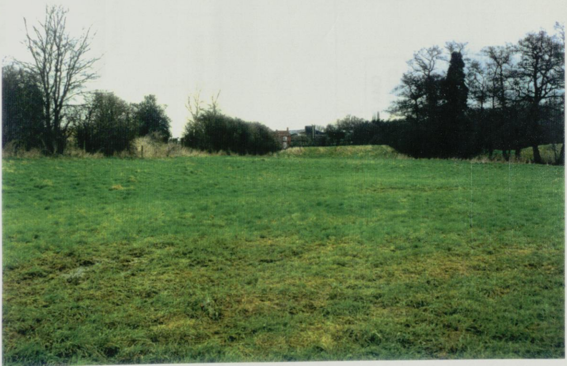
Northern Section of Cryfield Dam, viewed from the East
