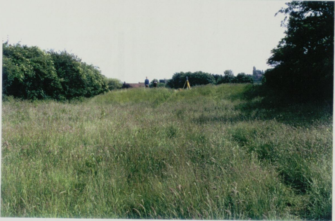
Northern section of Cryfield Dam, viewed from the West
