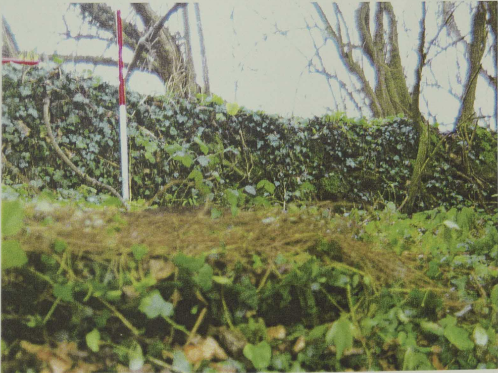
4. Photographing to show portion of sandstone wall that retains the leat.
