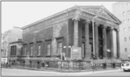
Elgin Place Congregational Church, Glasgow, now demolished.
