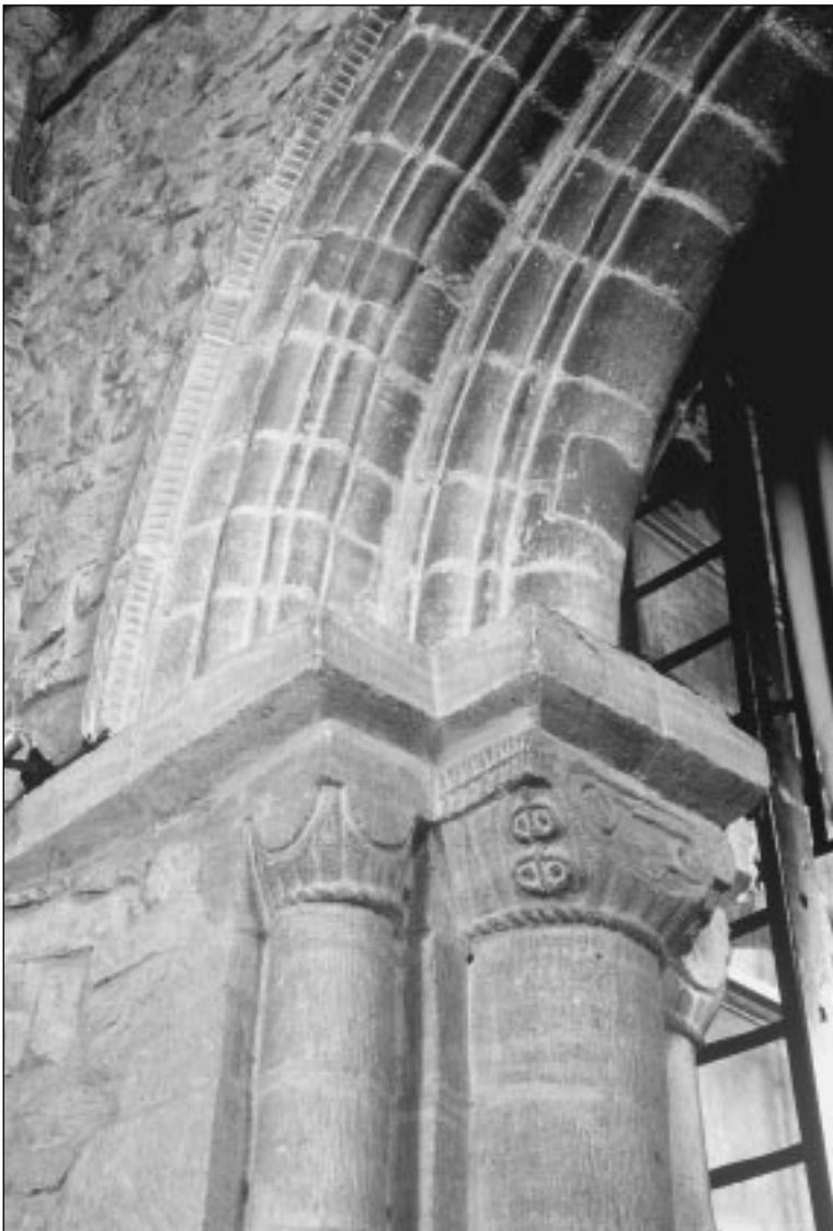
Fig. 13. Morcott, St Mary, arch to W tower, S capitals..
