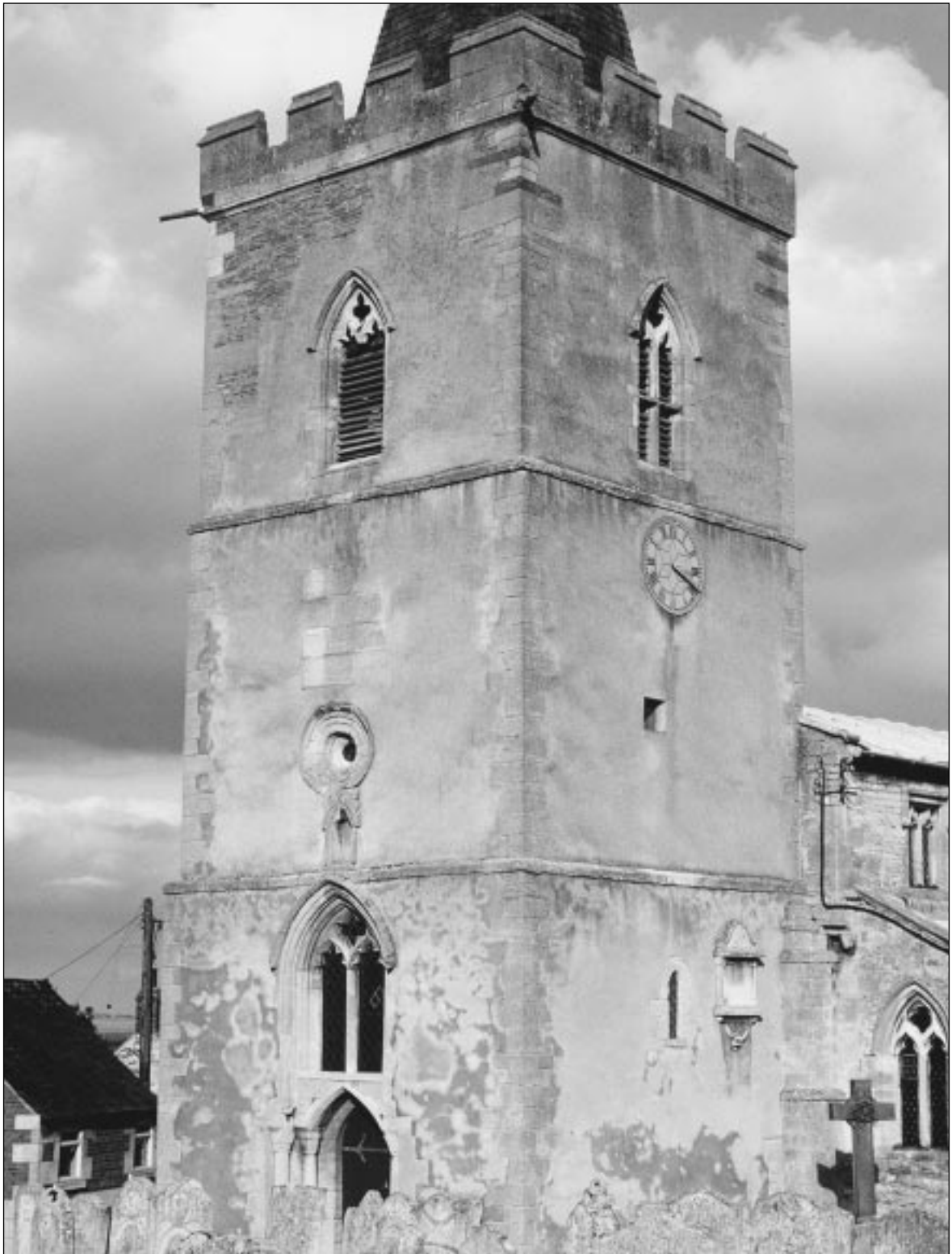
Fig. 7. Morcott, St Mary, W tower, from SW.
