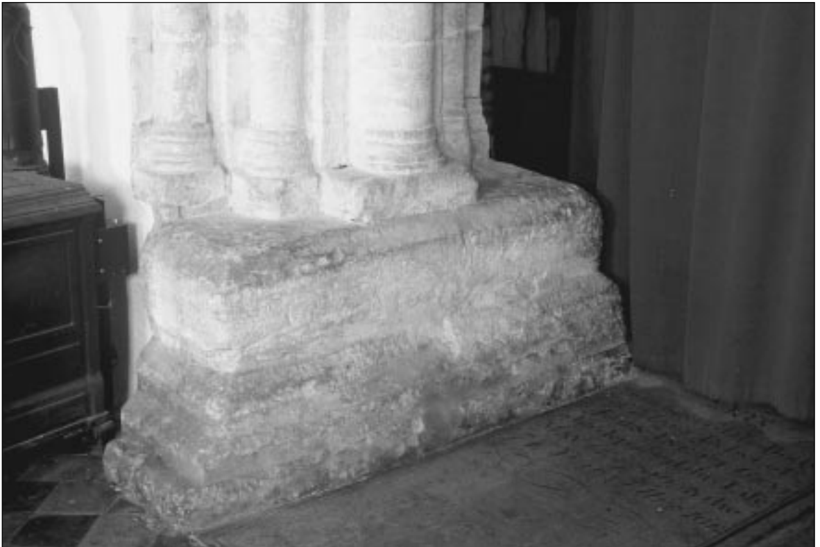
Fig. 4. Tixover, St Mary Magdalene, arch to W tower, N bases.
