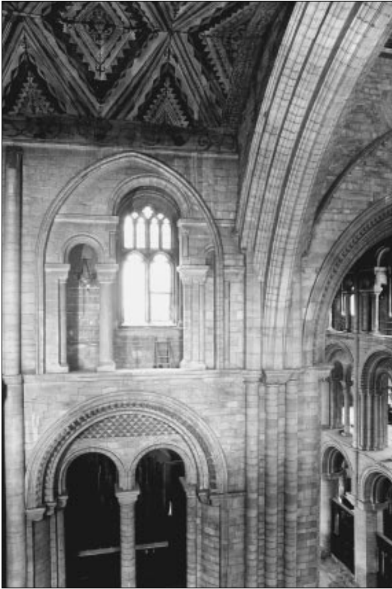
Fig. 1 Peterborough Cathedral, N nave clerestory, E bay.
