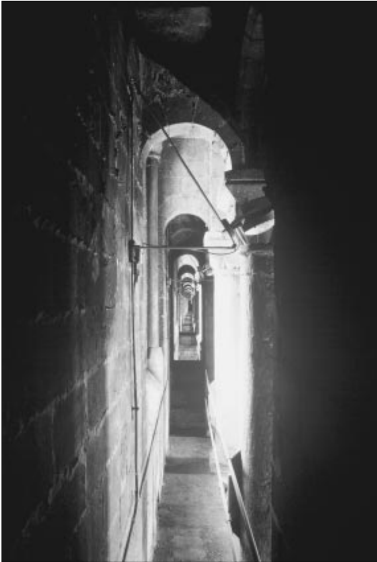
Fig. 7 Peterborough Cathedral, N nave clerestory, E bay.
