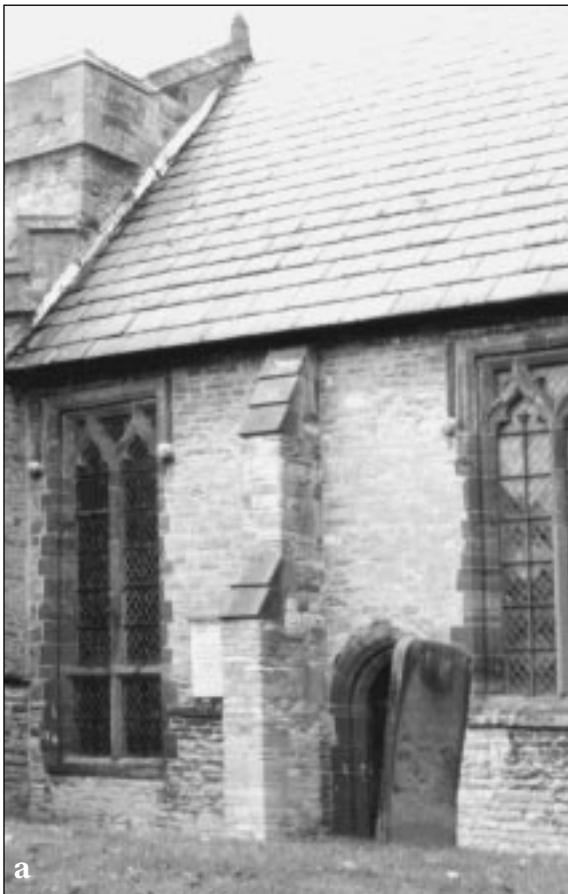
Fig. 4 St Mary's Grendon, Northamptonshire. Contemporary low side windows of differing form. a: south: low side window in both lights. b: north: low side window in one light. © Copyright English Heritage. NMR.
