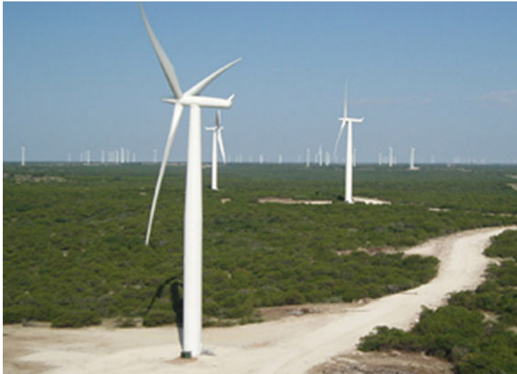
SWP 2.3-93 at Horse Hollow, USA (courtesy: Siemens Wind Power)
