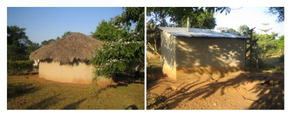
Figure 6: Thatched roof (left) and Iron Sheets roof construction (right). Source: The authors
