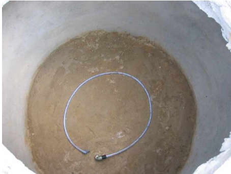
Figure 3 Drainage hose arrangement
