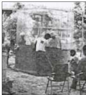
Partially rendered tank
