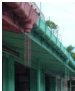
Extruded plastic gutters in Sri Lanka Note: Chains used to direct downflow
