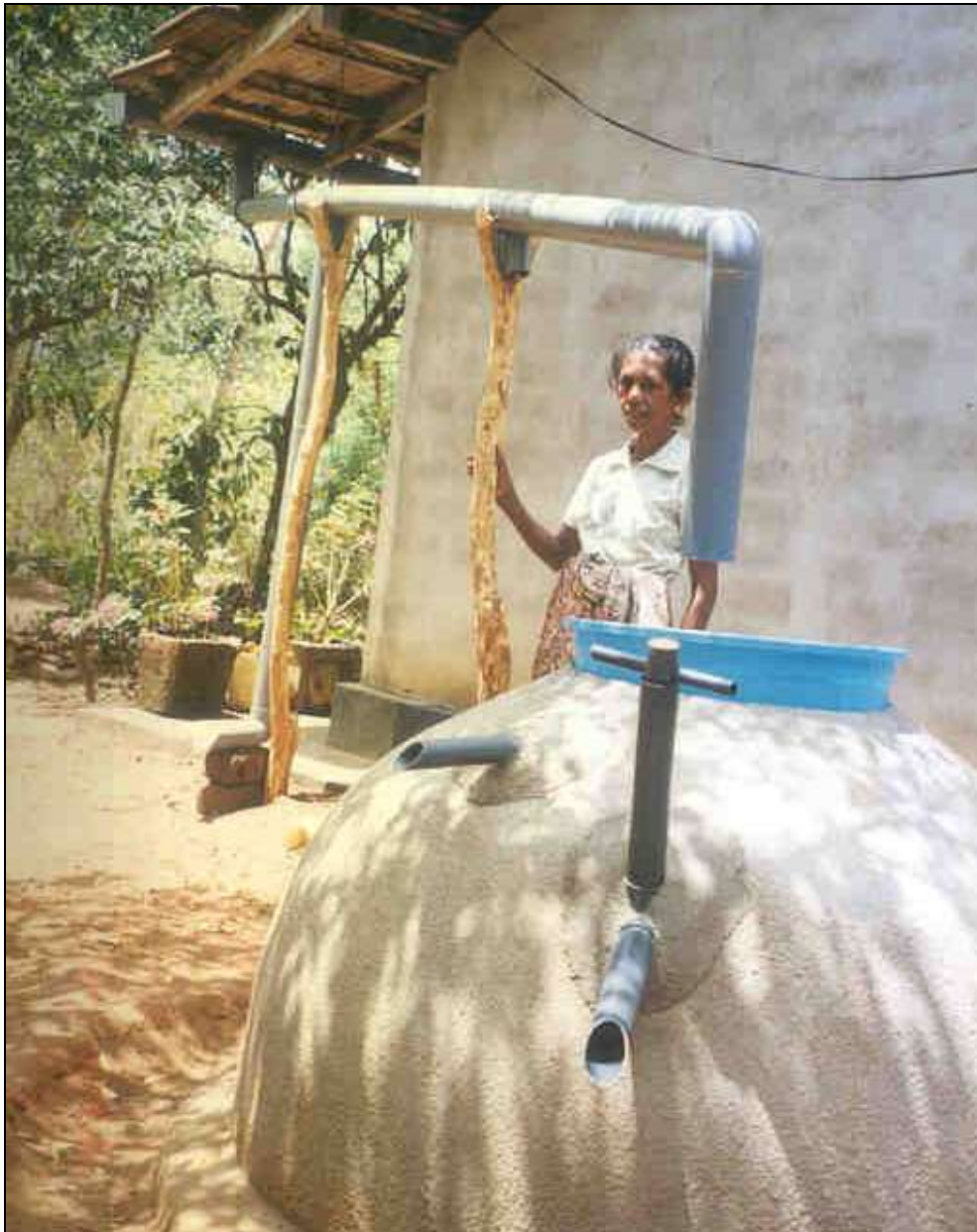
Figure 1.2: Roofwater harvesting system in a Sri Lanka
