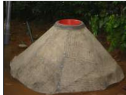
Good top seals and tar sheet cover used in Sri Lanka
