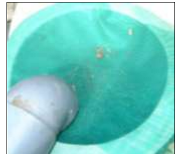
Coarse mesh leaf filter at tank entrance in Sri Lanka
