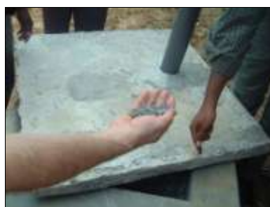
Filter media from a large gravel filter in Sri Lanka
