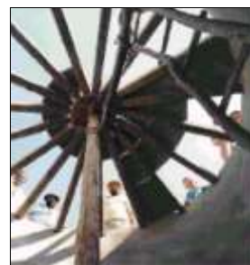
Precast roof plates being placed on a tank in Brazil [picture: [Gnadlinger, 1999]
