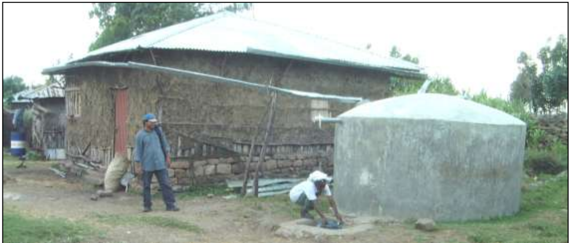
Figure 4.3: Wattle and daub dwelling in Ethiopia with large and expensive ferrocement tank
