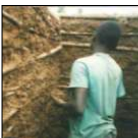
Daubing the walls
