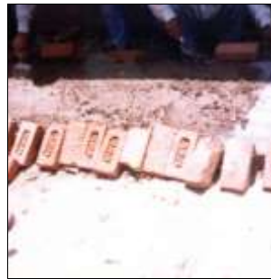
Laying mortar on mesh
