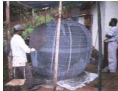
Partially rendered tank
