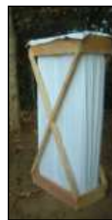
completed fabric tank
