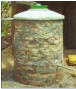
Burned brick tank in rural Uganda [Picture: V. Whitehead]
