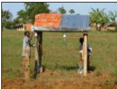
a. Tile and GI roofs
