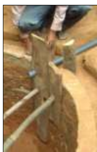
Shuttering for pump and overflow mounting
