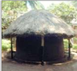
Finished 5m 3 tank
