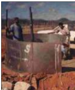
Screwing together the steel sheet form
