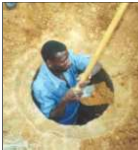
Digging the hole
