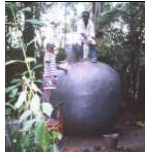
Finished tank [Pictures D. Rees]
