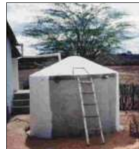
Finished tank being painted
