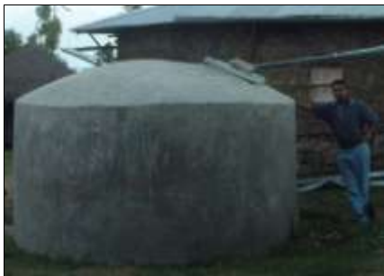
Household ferrocement tank in Ethiopia [Picture: S. Akhter]
