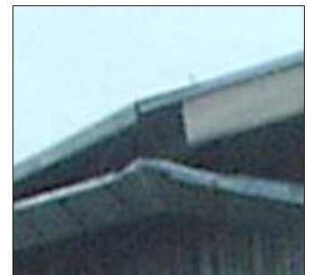
Vee shaped gutters with splash guard in Ethiopia
