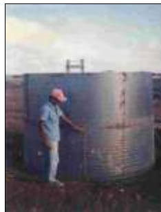
Steel sheet form, wrapped by wire mesh and galvanized wire
