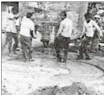
Moving the mould into place Note: pictures taken IRDC [1986]
