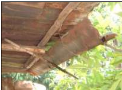
Ad-hoc mounting of vee shaped gutter using wires and roundwood in Ethiopia
