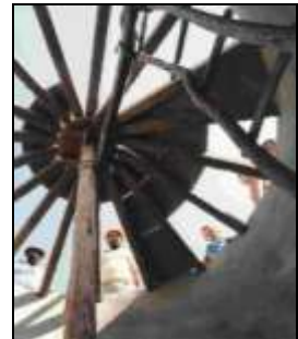
Installing the roof
