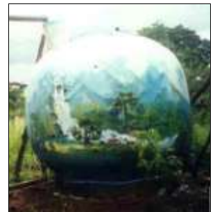
Ferrocement "pumpkin" tank in Sri Lanka [Picture: T. Ariyananda]
