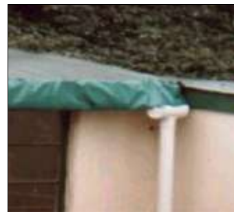
Experimental shade cloth gutters in South Africa [Picture Morgan [1998]]
