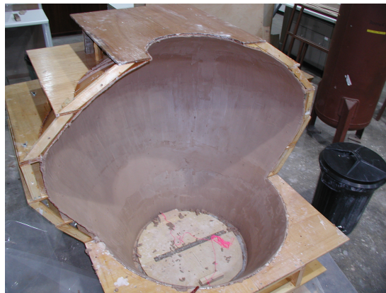
Figure 7.3: Application of mud coating to wooden tank mould
