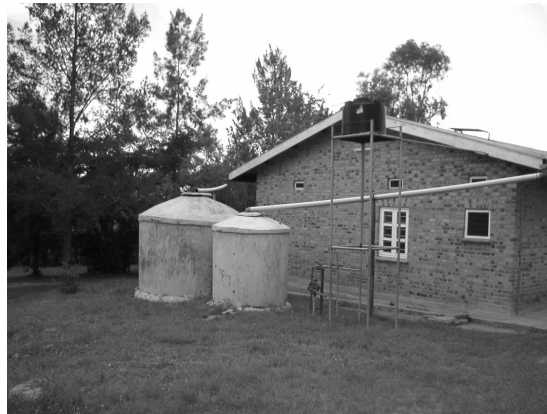
Figure 4.1: Example rainwater harvesting system
