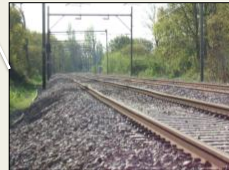
Hawkwell Railway embankment
