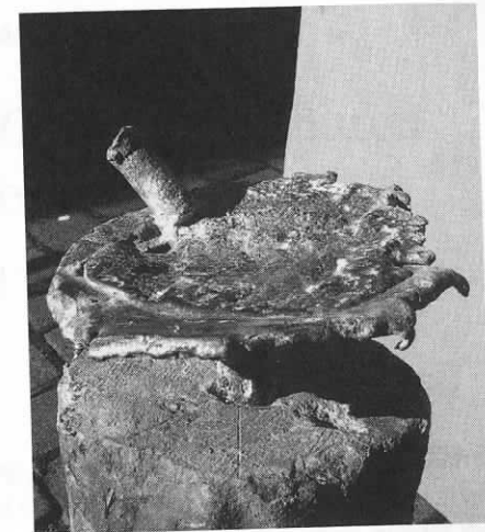
Figure 15.3 Limestone shaft from Lincoln Cathedral with partially dismantled lead joint. Note pouring hole on left (photo: author).
