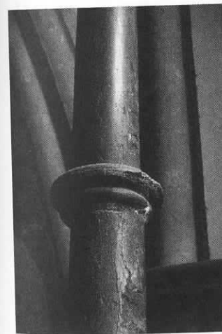
Figure 15.4 Rochester Cathedral presbytery; Purbeck shaft with poured lead joint and pouring hole evident on right (photo: author)
