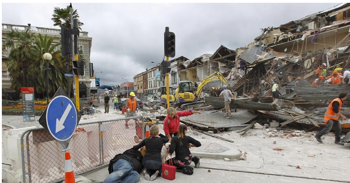
Figure 10: Photo of the destruction of the February 2011 Christchurch earthquake (BBC News 2011)
