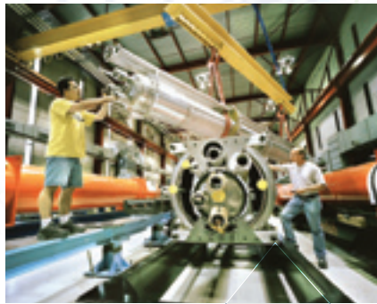
The LHC has some 5600 superconducting magnets installed around the collider ring, which is 27 km in circumference.
