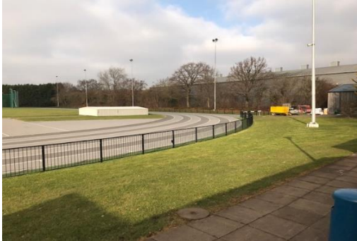
Photo taken towards the North of the site.
