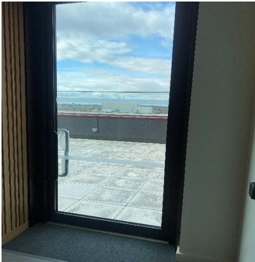
Main access door from lobby on fifth floor that and Salto access.
